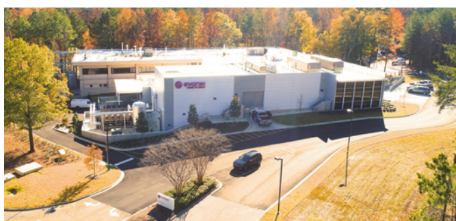
Evonik Birmingham Laboratories, Alabama, USA
